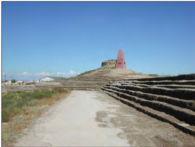
Kinney Dam looking north
